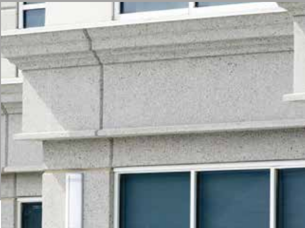
Medical Facility Salt Lake City, UT
